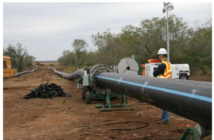
"Quality control and on-site testing were important issues for SAWS," said Radoszewski, "and would have been very costly to do for coated steel pipe. HDPE proved to be a leak-free material, with no cathodic protection required, leading to lower maintenance costs,
